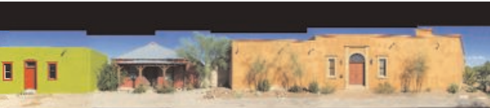
Newly constructed houses along Meyer Avenue resemble nearby 19th-century Sonoran-style row houses.
