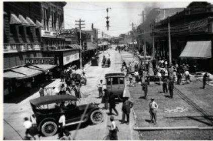
Workers pave street east of Scott Avenue, c. 1920
